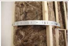
5) Insert the Dukta panels into the metal moulding and secure them by means of headless pins
